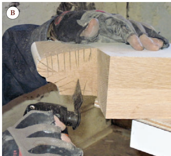
Figure 7. After scribing the replacement sills in place (A), the author used a multi-tool to kerf to the lines (B), then a chisel to remove the waste (C). A grinder with a carving blade was useful for matching the three-dimensional stone surface (D).
