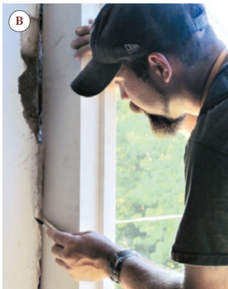
Figure 9. To provide a tight fit for the new interior casing, which would have to be installed from outside, the author temporarily positioned the replacement buck (A) and scribed an offset line on the plaster in the window well (B). He then removed the frame and cut the line with a grinder (C).
