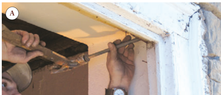
Figure 2. To remove a window frame, the author pounds out the peg securing the corner joint (A) and removes the side jamb (B). For windows whose jambs were in reasonable condition, only the sills were cut out (C).
