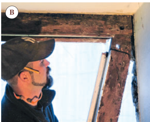
Figure 2. To remove a window frame, the author pounds out the peg securing the corner joint (A) and removes the side jamb (B). For windows whose jambs were in reasonable condition, only the sills were cut out (C).
