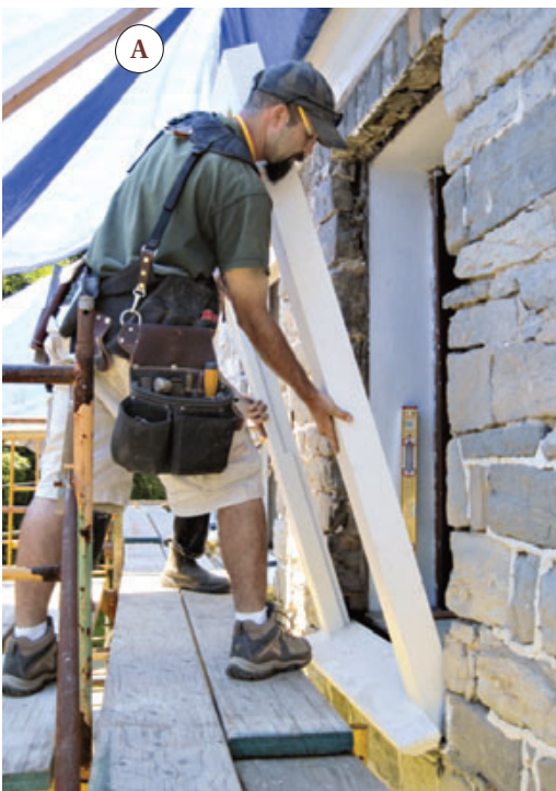
Figure 9. To provide a tight fit for the new interior casing, which would have to be installed from outside, the author temporarily positioned the replacement buck (A) and scribed an offset line on the plaster in the window well (B). He then removed the frame and cut the line with a grinder (C).
