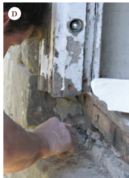
Figure 6. Before replacing the sills of the original window frames, the crew made sure the head and jambs were in plane (A), then clamped them in place (B) and drilled the holes for the epoxy anchors (C). With the jamb bolted in place, the mason repairs the window well before the primed sill is installed (D).
