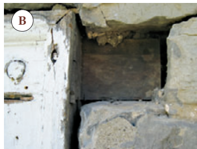
Figure 1. The old window frames were mortise-and-tenoned together (A). The top jambs had “ears” — extensions that allowed the window frame to be mortared securely in place (B). Where the stone got in the way, the original carpenters cut off the ears and inserted wood pegs for keying the bucks to the masonry (C).
