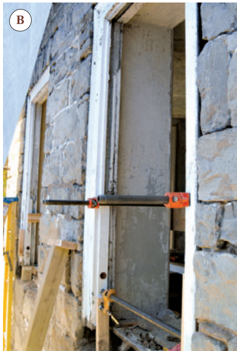
Figure 6. Before replacing the sills of the original window frames, the crew made sure the head and jambs were in plane (A), then clamped them in place (B) and drilled the holes for the epoxy anchors (C). With the jamb bolted in place, the mason repairs the window well before the primed sill is installed (D).
