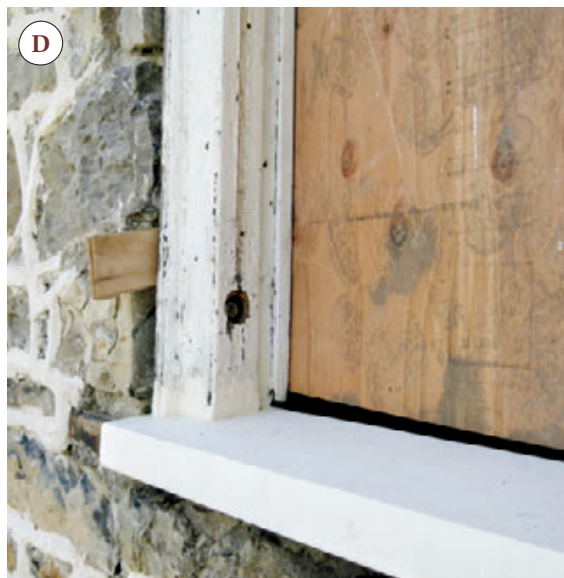
Figure 8. Threaded rod glued in holes in the ends of the replacement sills (A, B) served the same purpose as the wood extension “ears” on the original sills — providing anchorage in the masonry (C). The old jams were first epoxied to the stone, and the new sills attached from the bottom with lag screws driven at an angle from beneath (D).
