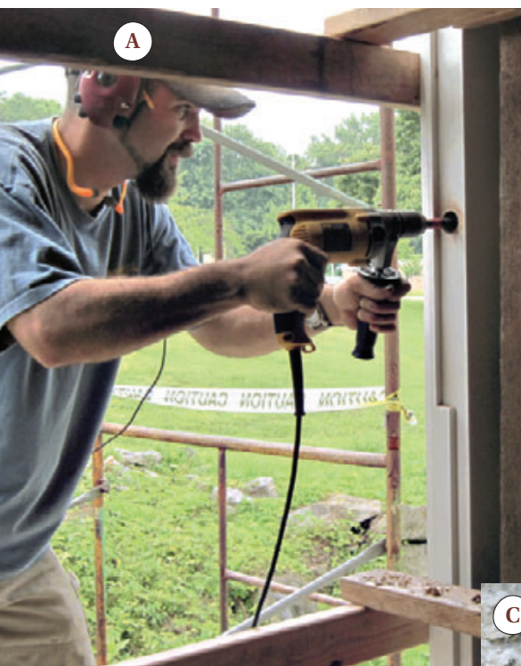
Figure 5. To attach a new wood window frame to the stone with threaded rod, the author first drilled a hole large enough to accommodate the washer and nut, using a wood countersink (A). To avoid ruining the bit, he continued drilling through the wood with a 1/2-inch masonry bit until he hit the stone. Then, with the frame out of the way, he continued drilling with a 5/8-inch masonry bit, making a hole large enough for the 1/2-inch rod and the epoxy (B). To ensure a good bond, he cleaned the hole with a wire brush (C) and compressed air (D).
