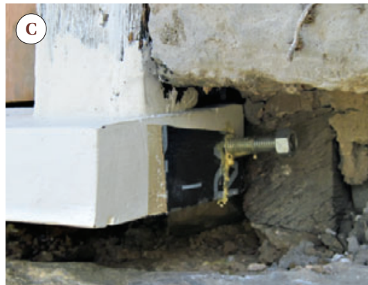
Figure 8. Threaded rod glued in holes in the ends of the replacement sills (A, B) served the same purpose as the wood extension “ears” on the original sills — providing anchorage in the masonry (C). The old jams were first epoxied to the stone, and the new sills attached from the bottom with lag screws driven at an angle from beneath (D).
