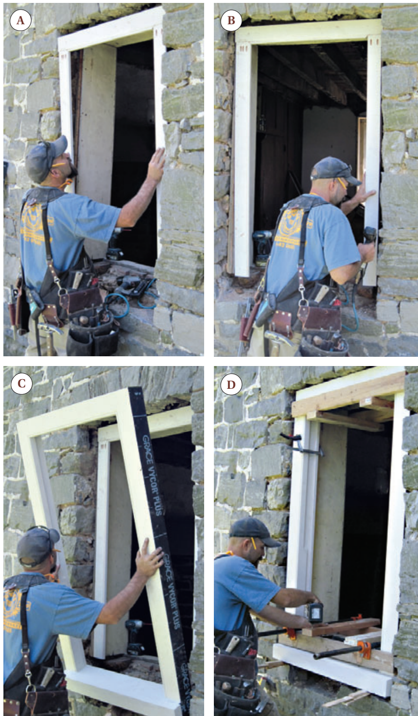
Figure 10. Before the new window frame could be installed, the casing had to be pocket-screwed together (A), then positioned from outside and tacked into place (B). The window frame, protected on all four sides with peel-and-stick membrane, was then set in the opening (C) and secured in its final position in preparation for installation of the epoxy anchors (D).
