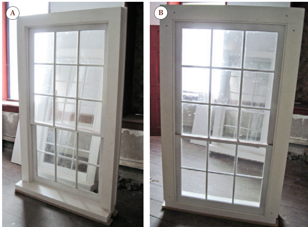
Figure 3. The replacement units (A) came with beaded interior casings tacked into place (B). The replacement sills matched the profile of the originals (C); they came primed and cut to length, but the carpenters had to scribe and cut out the returns on site.
